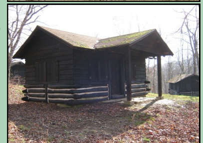
Historic (top) and modern (bottom) photos of CCC cabins at Raccoon Creek State Park. Using a log and frame construction, the architecture of these cabins was unique to Raccoon Creek State Park.
